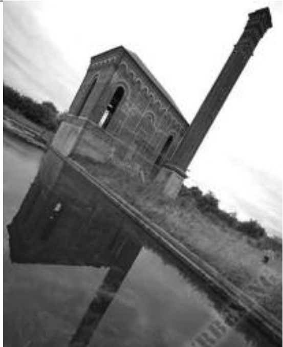
Bracebridge Pumping Station. Image © tims, www.urbexing.co.uk
